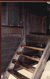
Stairs down to the bathroom
